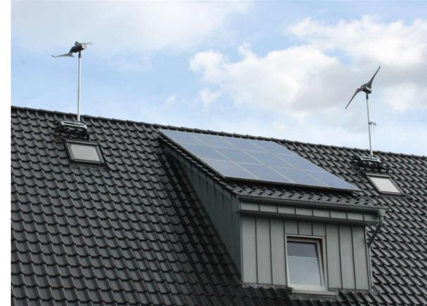
Decoupled roof-top mounted SkyWind NG turbines
