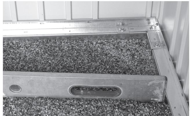
**(GB)** Fill up the bottom with gravel, so that the heads of the soil anchors disappear. Level the surface again horizontal. Now insert the floor plate(s) as shown. The floor plates are connected by the aluminium-profile(s). The floor plates must not screwed up as they are positioned exactly within the base frame.
