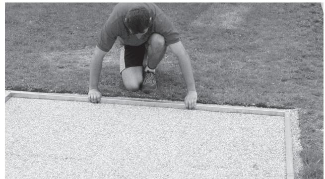
**(GB)** Place the base frame onto the gravel bed and put the shed onto the base frame. Connect the shed together with the clamping angles\* (z-shape) by means of the hexagonal self tapping screws\* + washers\* to the base frame. For good orders sake check the base frame with regard to rectangularity (equal diagonal measure). Now anchor the base frame as shown by means of the soil anchors\*. (\*= part of the base frame set)
